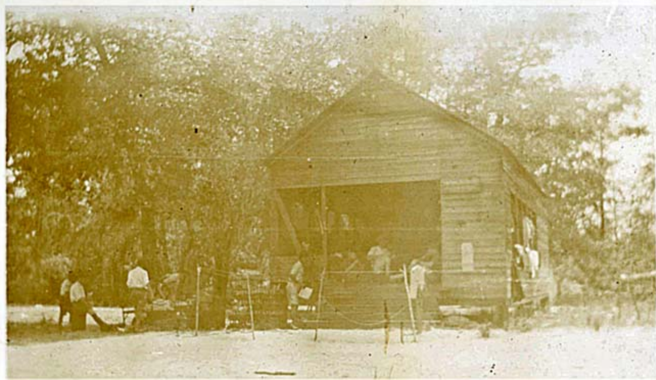
Headquarters and also canteen.
